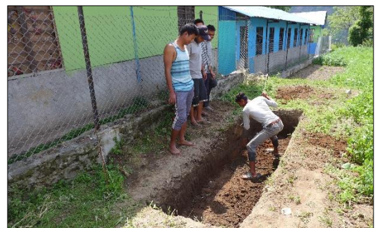
Trench being dig. ©CRAterre, Sindhupalchok, Nepal
