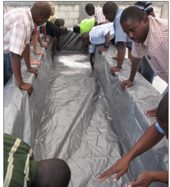
Waterproofing of a wooden tank using a tarpaulin. ©CRATERRE, Haiti
