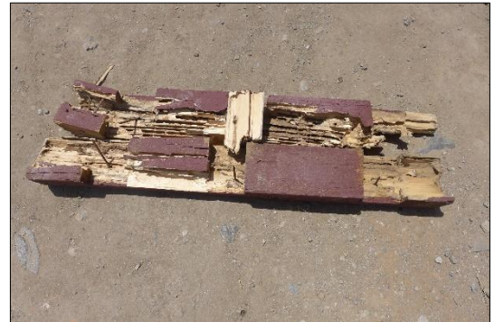
This wood piece that was preventively painted for protecting it was completely eaten by termites within the course of 8 months.
